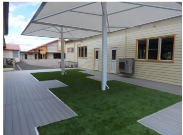
The new covered open air reading area
