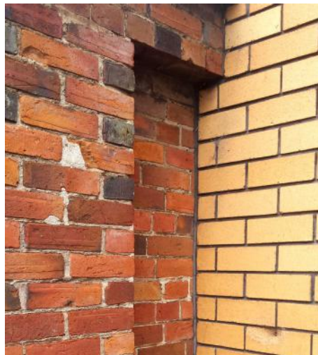
1880s meets 1980s brickwork at Hill Street reservoir
